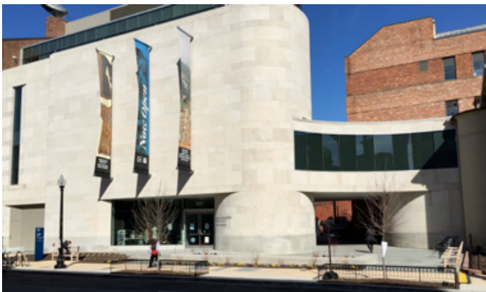
1. Exterior of the new Textile Museum
